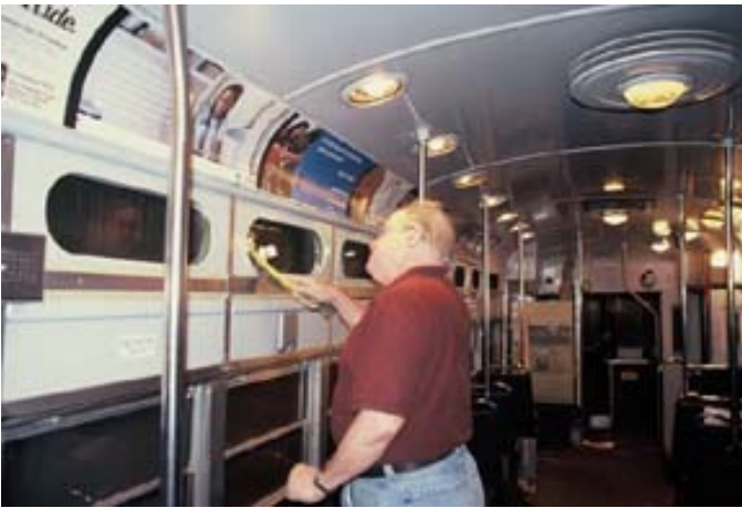
2006 – Interior work progresses. All loose paint and scale was removed and the new paint was computer matched to the old. A faulty front door relay was replaced as well.
