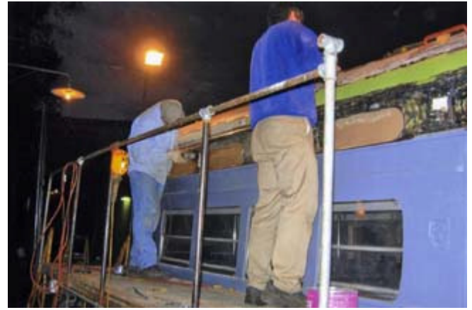
November 2008 – Working under the lights to keep the project moving.
