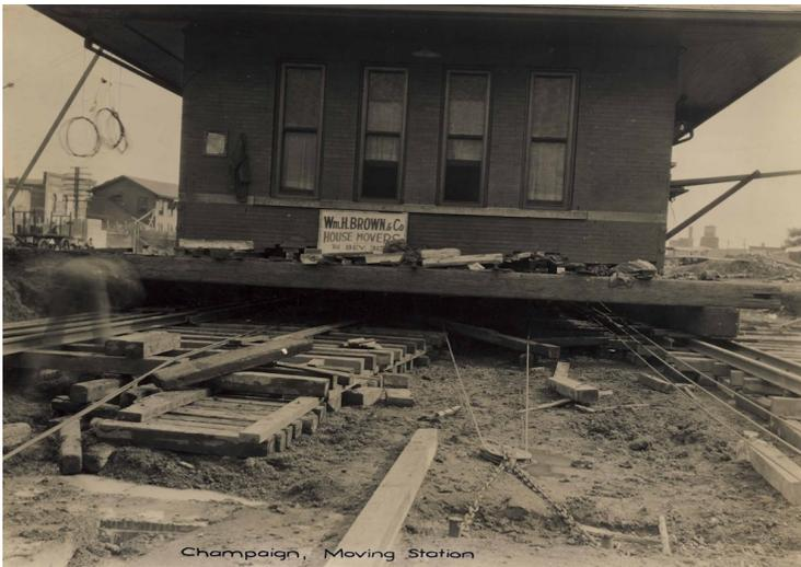
Another view of the rail system set up to move the station north. Photo courtesy of the Illinois Central Railroad
