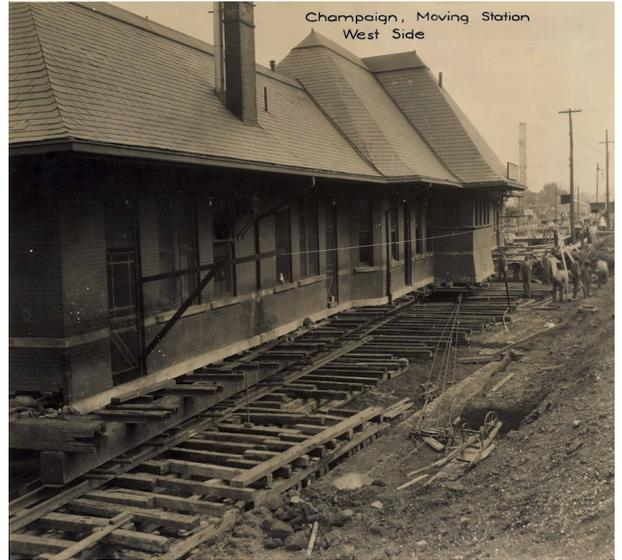
The depot is pulled north by a series of rails and pulley's.
