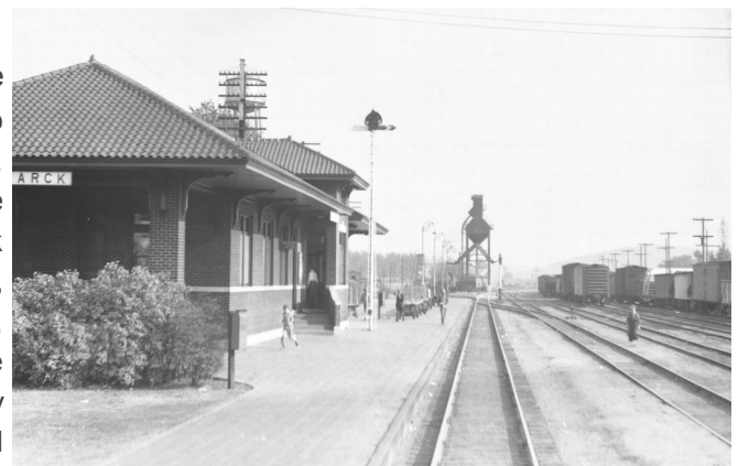
Bismarck, MO—Built by Missouri Pacific in 1916. Photo courtesy of the John Barriger Railroad Library
