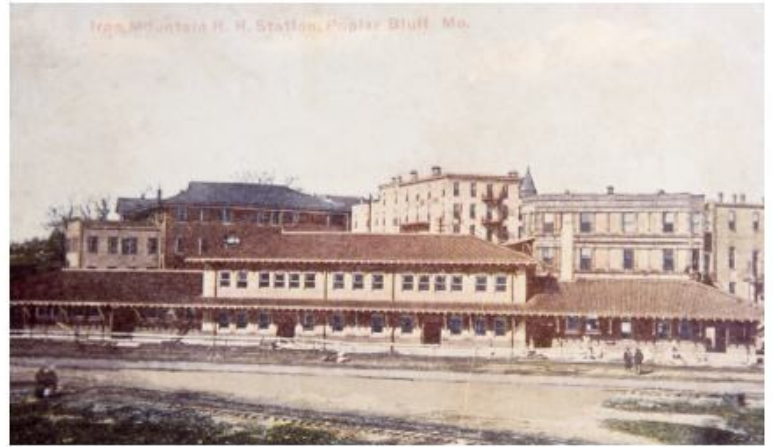
Poplar Bluff, MO—St. Louis & Iron Mountain Railroad Station. — courtesy MPHS Archives
